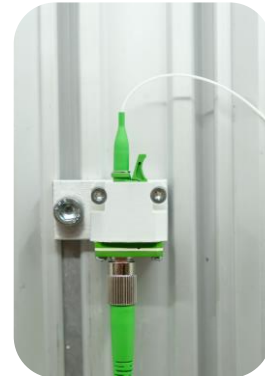
6. Insert the new connector and make sure it clicks in place
